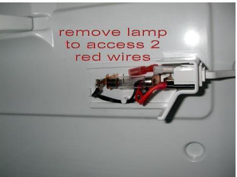
3. I then attached a female connector to the wire close to the switch and a male connector to the wire that goes through the hole in the refrigerator. I covered the male connector with electrical tape. If I need to use the heater in the future, I just join the two connectors.
