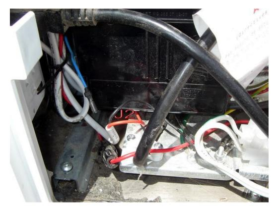
2. I then removed the light cover in the refrigerator and found the two red wires attached to the light switch. I pulled them out as far as I could and cut the one that was a larger diameter than the one identified in step 1.
