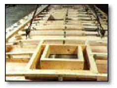
This construction is similar to the way houses are built in that there is a frame of wood or metal that provides the structural form. Paneling is stapled and/or glued to the inside and aluminum siding is then stapled to the exterior framework. Insulation is contained within the cavities of the framing members and is normally fiberglass wool. The various window and door openings, and all the appliance access openings are framed with wood members as part of the structure.
