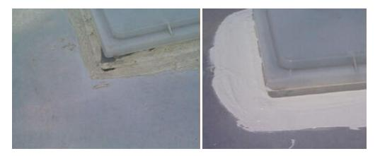
The roof coat has been re-newed and this vent is again sealed.
