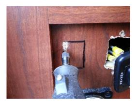
The hole cut, now I am ready to run the wire. I checked before hand and I do have a clear path from the convenience panel down to the switch site. It helped to remove the furnace diffuser to fish the wire. I need 3 conductor wire; one wire is the hot, the other two are the switched lines. I happened to have a 5 conductor bonded wire. I used it – this would give me two wires for spares for whatever else I might want to add in the future.
