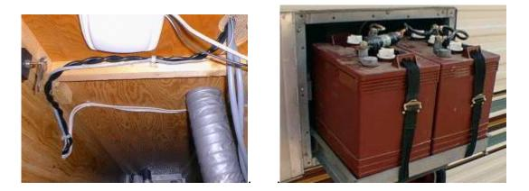
Once all that was done, I ran some wiring for the remote on/off switch for the inverter function. This lets you disable the inverter when it's not needed. You could really leave it on all the time, but the inverter does draw about 1/2 amp in standby (when there is no load on the AC outputs) so I would rather turn it off when not in use to save power. I mounted the switch next to my monitor panel (more on the monitor panel later...) as seen here.
