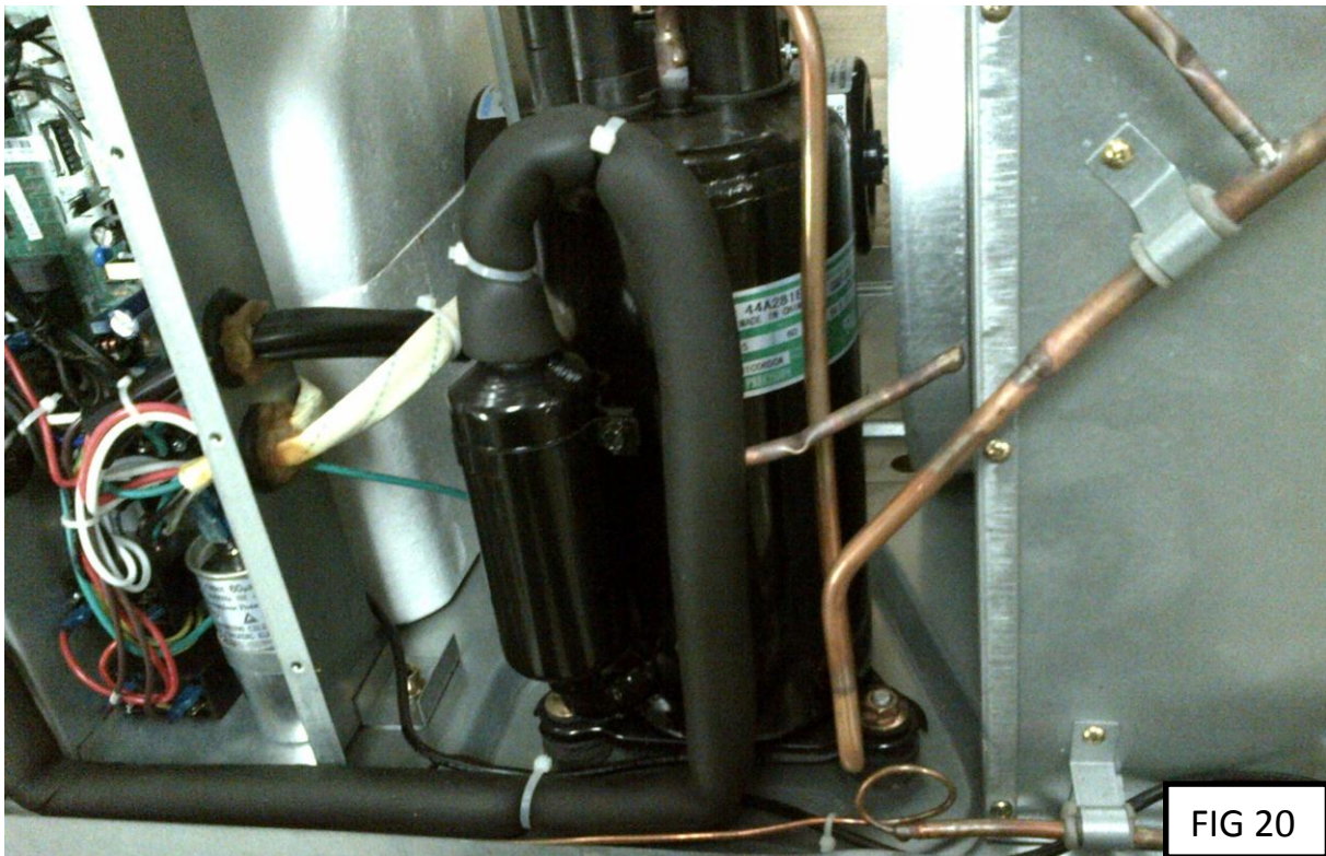
View of Compressor inside Rooftop Unit
