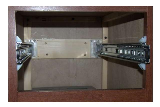
I found it easiest to measure for center on the front face frame, mount the front guides, then used a level on the slides to get the rear sockets positioned correctly. Of course this technique needs the trailer to be level as well.
